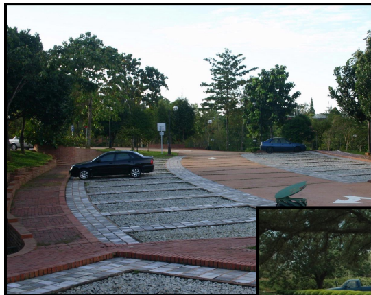
Left: Installing permeable pavers in place of concrete or pavement allows for greater stormwater infiltration and helps minimize root/pavement conflicts near plantings. W. Fountain, Univ. of Kentucky, Bugwood.org
