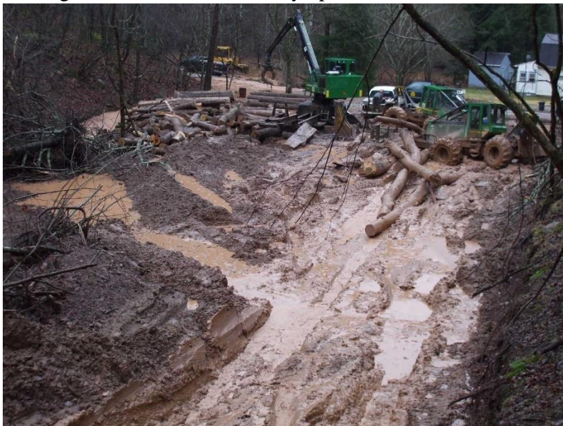
Figure 4.1: Extreme Sedimentation due to poor logging practices. (Source: WVDOF)
