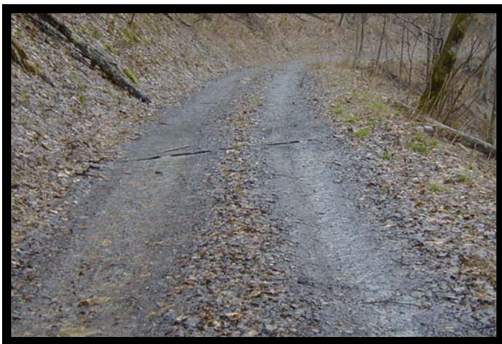
Open-top pipe culvert.
