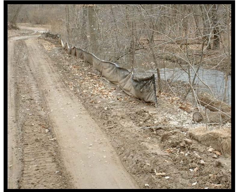
Silt-fence application.
