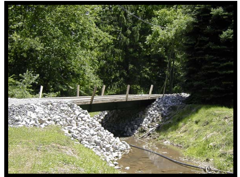
Portable temporary bridge.
